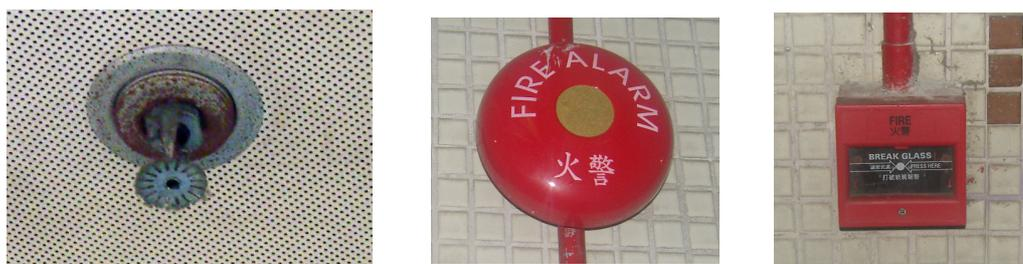
Figure 1.2 Sprinkler head (left); Alarm gong (mid); Break glass (right)
